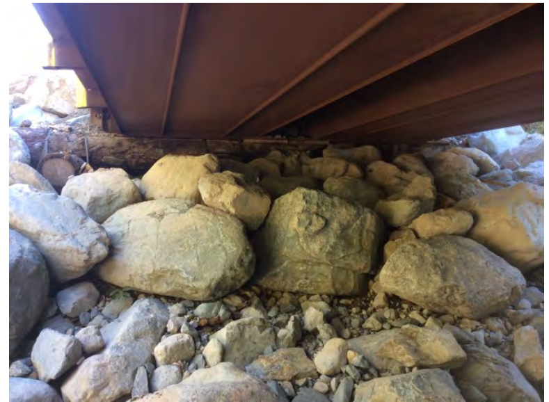
Right Bank Abutment when facing downstream
