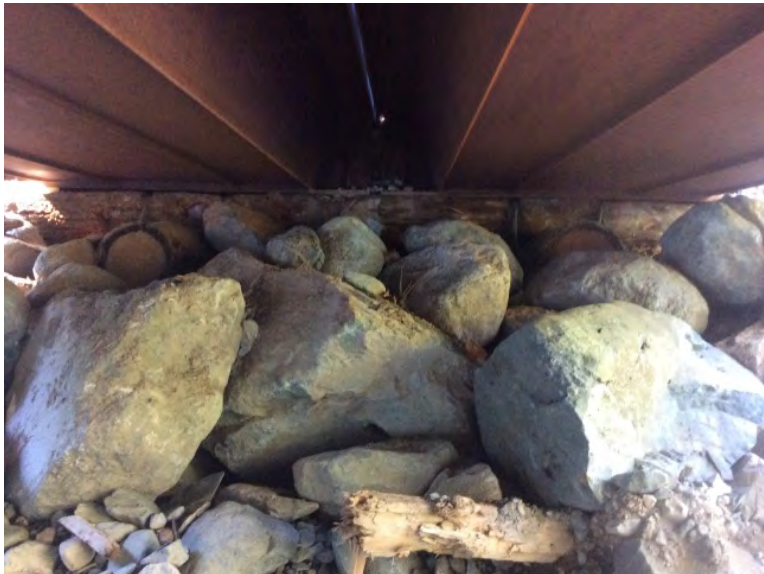
Left Bank Abutment when facing downstream
