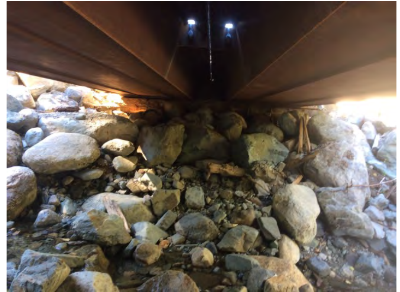
Left Bank Abutment when facing downstream
