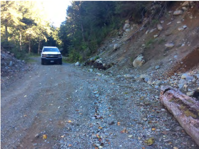
Approach from Left Bank when facing downstream — ditch line needs redefining as is eroded no road surface on woods side
