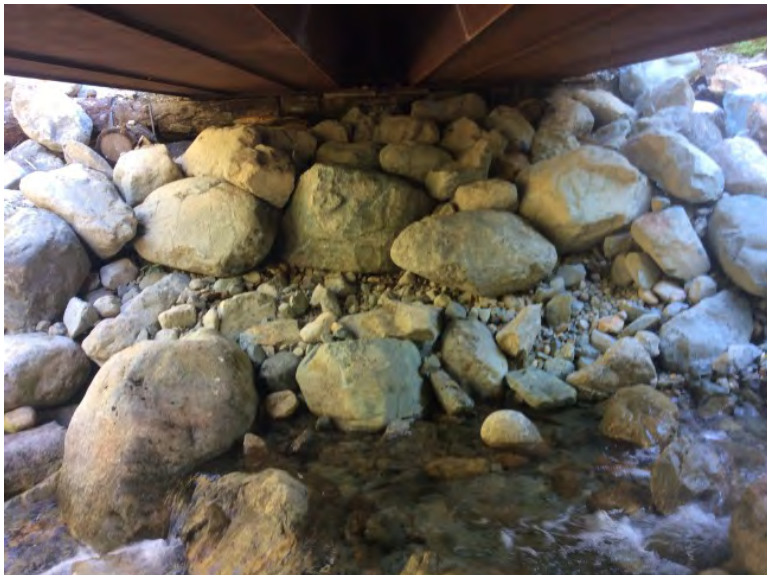
Right Bank Abutment when facing downstream
